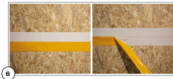
2. Fold the border of the adjacent carpet upwards to the side and stick the adhesive tape right next to the previously glued adhesive tape. Also release the yellow guard band. (Pic. 6)
