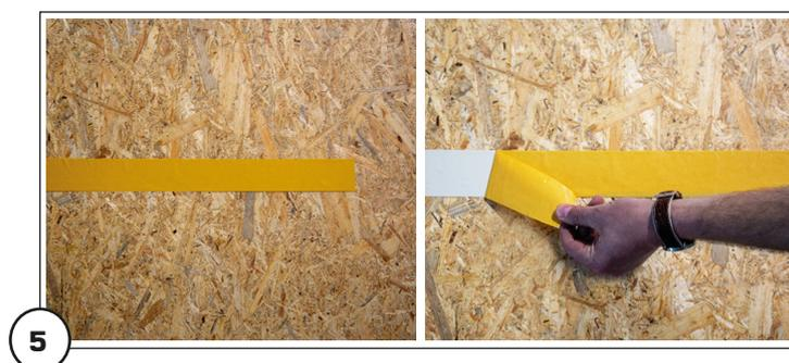
1. Fold up one long side of the carpet to the side and stick the adhesive tape on the subconstruction. Release the yellow guard band. (Pic. 5)
